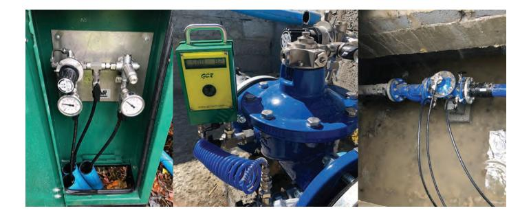
PRV pilots can be controlled mechanically, as at Rathgormack, or remotely using electronic control systems such as SCADA. AVK's acquisition of Italian valves specialist ACMO has broadened AVK's SMART network offer and greatly enhanced AVK Group's ability to develop automatic valve control systems.
