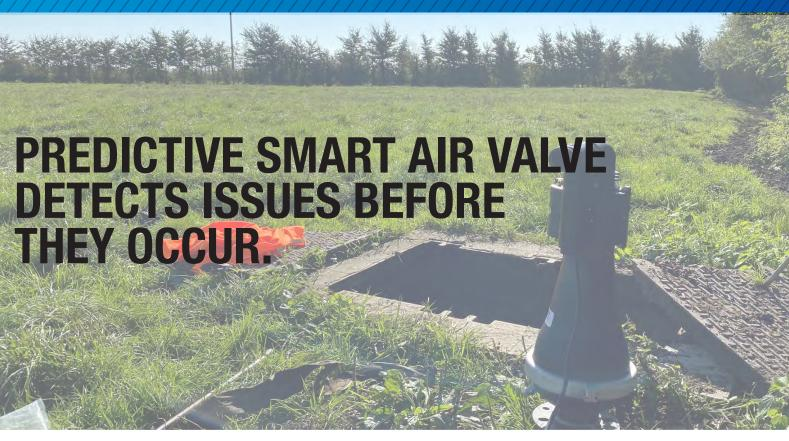
Wessex Water has trialled an AVK UK wastewater smart air valve on its network near Weston-super-Mare. An alert triggered by the air valve ensured Wessex Water was able to respond quickly to flooding in the valve chamber which eliminated the possibility of sewage entering the adjacent water courses.
