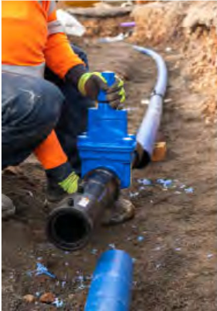
Image above shows the installation of a Series 36/89 Gate Valve with PE Pipe Ends
